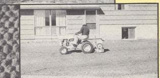
With blade floating between Grid Roller and tractor wheels, it can be raised or lowered by the pitch control for a perfect levelling job.
